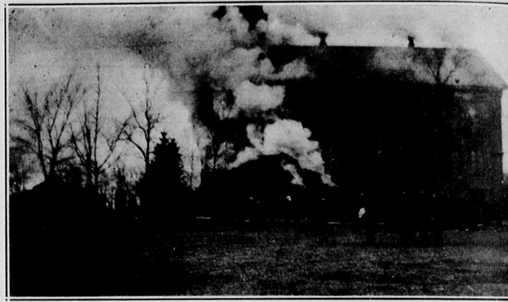
The local fire department poured a lot of water around this building in their tests and coupling contests this summer, but back in 1898 or '99 it really needed water. It's the South church in flames forty years ago.
