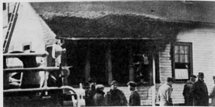
Photo by Donald Surette Fire which damaged a Bellevue road home a week ago, caused by a gasoline stove explosion.
