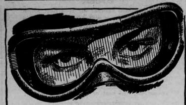
EYELIDS CAN FREEZE SHUT IN HIGH-ALTITUDE FLYING. SO GENERAL ELECTRIC ENGINEERS DEVELOPED ELECTRICALLY HEATED GOGGLES. FINE WIRES ARE IMBEDDED IN PLASTIC LENSES. G.E. ALSO MAKES ELECTRI-CALLY HEATED FLYING SUITS, GLOVES, SHOES, CASUALTY BLANKETS.
