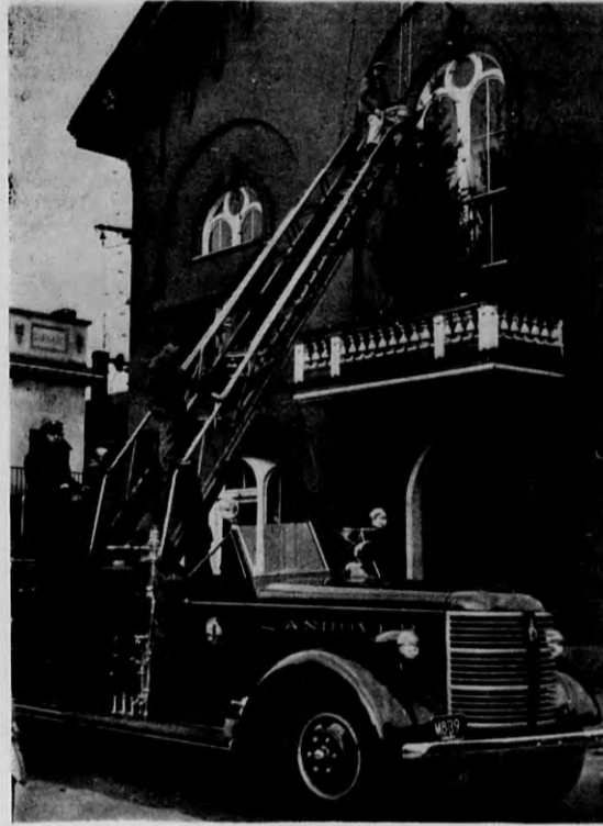
Getting ready for Yuletide, electricians enlist the aid of firemen and the ladder truck to decorate the front of the Town House with Christmas greens and lights. Leo Parsons is at the top of the ladder, Dale Webster is about to ascend, while fireman John T. Cole operates the "big stick."
