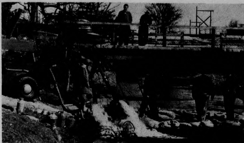
When a 16-inch water main broke last week in the bed of the Shawsheen river at Central street, workmen had to throw a coffer dam about the section of damaged pipe before repairs could be started. The brush fire truck and an auxiliary pumper from the central fire station were brought into use to pump water from the enclosure so employees of the board of public works could get to the bottom of the river. Photo of the scene shows George Williams, fireman off duty, and Timothy Daley, on the bridge. Below, Alexander H. Henderson, new member of the B. P. W., and Supt. Edward R. Lawson, standing on bank; others left to right, Stanley Chlebowski, foreman, Henry Burbine and Don Gillispie of the B. P. W. (Look Photo)
