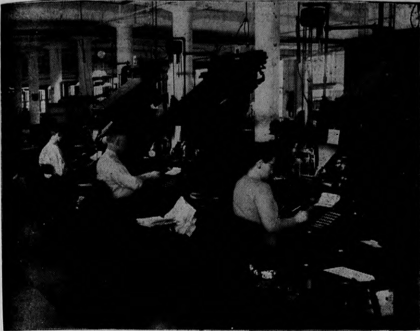
The linotype machines which economically and accurately set your copy in a minimum amount of time. These machines have a wide variety of type faces and in addition hand set type is available in numerous fonts to fit the needs of any style of printing.
