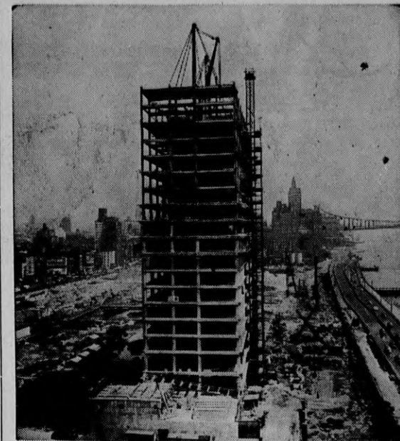
Steelwork on eighteen of the 39 stories of the United Nations Secretariat building in mid-Manhattan, New York, was completed in July when this picture was taken. A contract was signed by U.N. and the American Bridge Company for the furnishing and erection of structural steel for the meeting hall area of the Permanent Headquarters. The contract calls for 10,500 tons of structural steel at a cost of $2,225,000. Delivery is to be made by next October, and erection is expected to be completed by April or May 1950.
