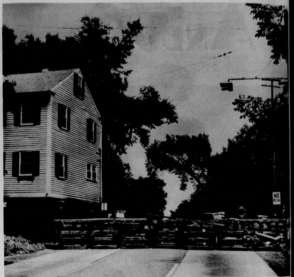
Moving one of Andover's old landmarks to make room for the new Phillips academy gym necessitates a trip across Route 28 on S. Main st., on this trestle. Once known as the Comstock house and now the residence of Leonard F. James, academy instructor and Townsman columnist now in Europe, it was moved a distance of nearly half a mile from Highland road to Hidden field. (Look Photo)
