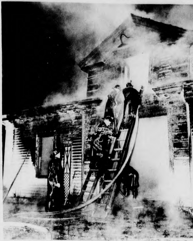
Firemen taking water lines into the flaming barn on the property of Ronald H. Sherman 66 Central st., Friday night. Shortly after this photo was made part of the roof collapsed endangering the lives of some of the men here pictured who had entered the building, and others who were working on the ground floor. (Look Photo)
