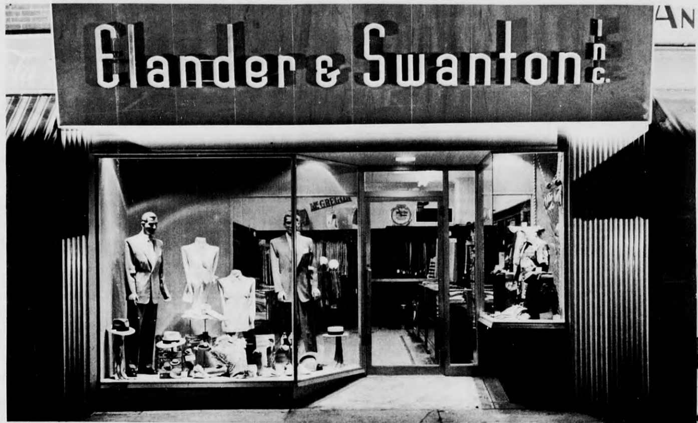
The new look at Elander & Swanton's. Pictured above is the new aluminum alloy and glass store front providing a bright new view of displays. To the right, the newly redecorated interior featuring new lighting and air-conditioning for shopping ease and comfort.
