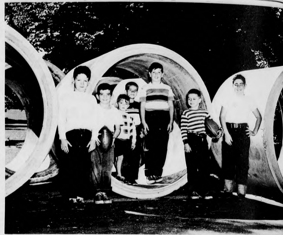
The large sections of reinforced concrete pipe that adorn one side of Chestnut street near the park are being used by the board of public works to enclose Rogers brook from Chestnut street southerly for a distance of 144 feet and are quite an attraction for youngsters. Each section is five feet in diameter and weighs two-and-one-half tons. In the photo are, from left to right, Jimmy Williams, Norman Wallace, Richard McIntyre, Bobby Mauck, Dennis Porter, "Bruby" Porter and "Butch" McIntyre.
