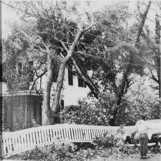
Historic elms, shading Barnard Arms on High street, shown against house where they were blown by wind. (Look Photo)
