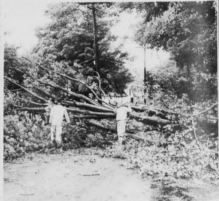
Clearing away large maple trees that had toppled across Lowell street near Canterbury after the storm. (Look Photo)
