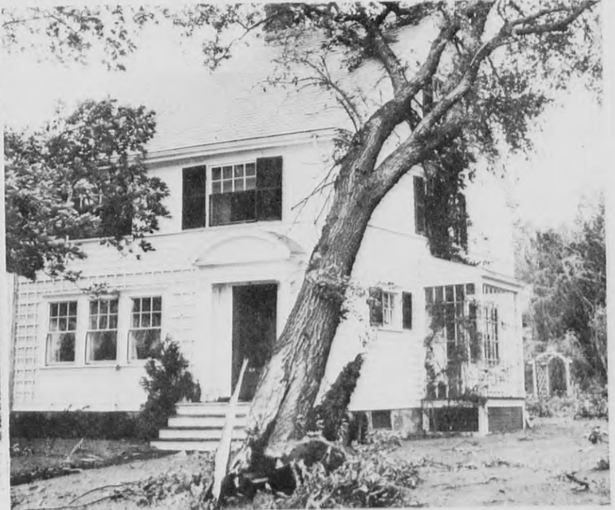
Ripped away from its base this giant tree fell on the house of Chester Blanchard at 64 Haverhill st., in Shawsheen. (Look Photo)
