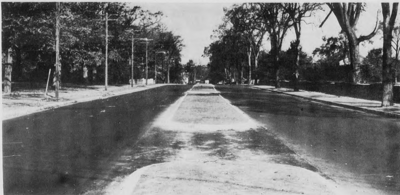
Elimination of a traffic hazard at the junction of School, Wheeler and Main streets has been completed with this new divided highway on Main street at the Phillips academy campus. The lane on the right was once a grass plot which has been removed to widen the road and facilitate the flow of Route 28 traffic which passes over this street. View shows street looking toward the square. (Look Photo)
