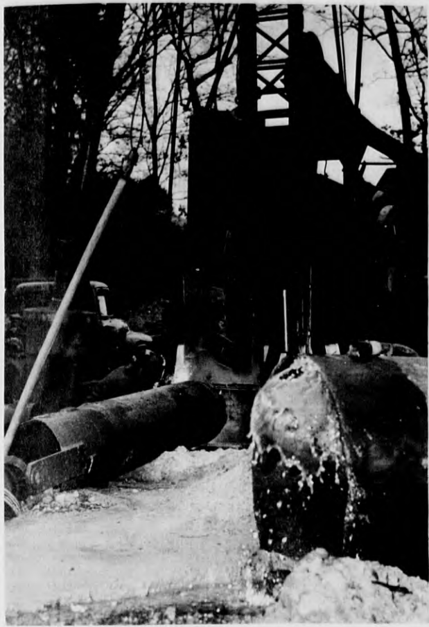
BALLARDVALE TEST WELL -- Installing the casing for the permanent well in Ballardvale kept workmen busy last week: They should be moving soon to the Abbot well, according to Water Dept. Supt. Donald Bassett. (Leone)
