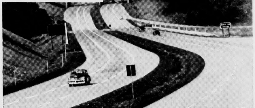
This new-type concrete road will last 50 years . . . and more.
