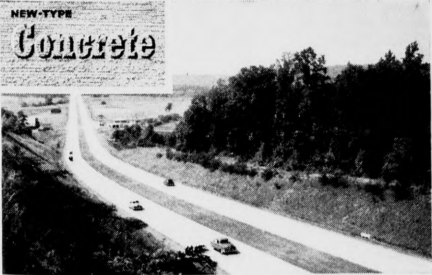
This new-type concrete road is smooth, quiet and comfortable
