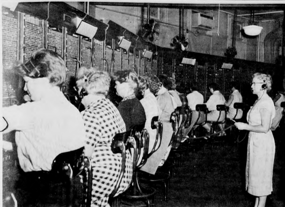
SOON, JUST A MEMORY - The busy telephone switchboard in the Musgrove Building will soon be only a memory, as conversion to the dial system takes place Sunday morning. Here, Mrs. Ethel Sullivan, chief operator, looks over a section of the switchboard as operators keep busy with the normal routine. Most operators, she said, are being transferred to other offices of their choice. (Staff Photo)
