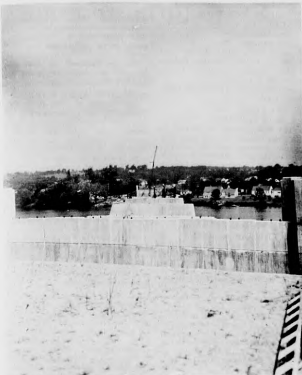
IN THE DISTANCE - Taken from the bank of the Merrimack, at the Andover end of the new bridge for Route 28, this photo shows the progress of the bridge project. Work started from the Methuen side, with a giant crane lifting multi-ton steel girders to their proper position atop the abutments. (Staff Photo)
