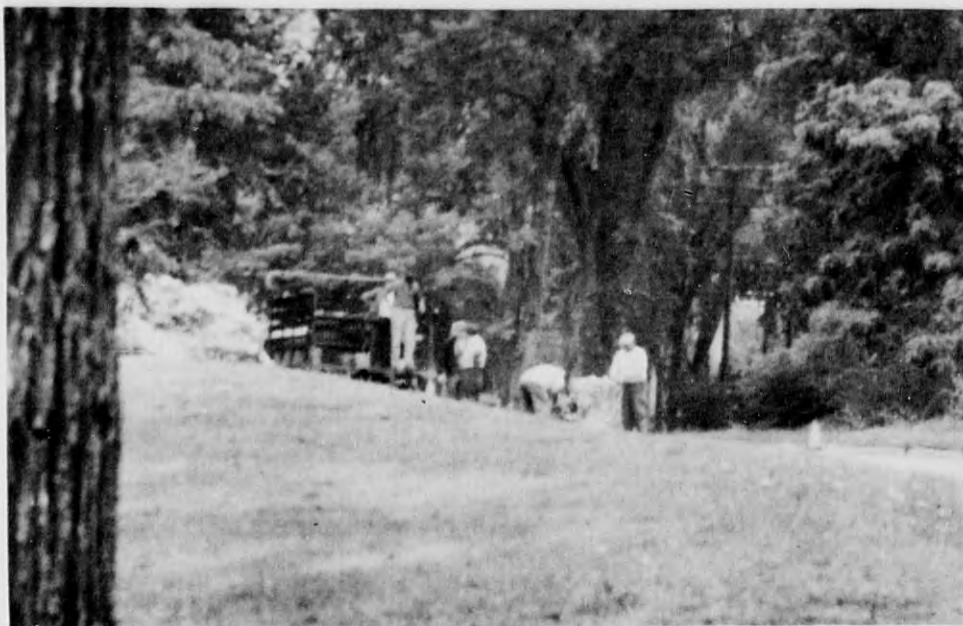
WORKING ON THE HIGHWAY — Six of an 12-man crew painting stripes along Route 28 last Friday were photographed as they paused in their labors. During the time they painted, one man ran the machine, which is being filled with paint in this picture. Three others walked beside him; one drove a truck with a passenger in the cab; while several rode in the rear of the truck. One of these men sat on the tailgate, putting markers down along the road. One walked ahead of the procession, using a red flag to warn motorists. (Staff Photo)
