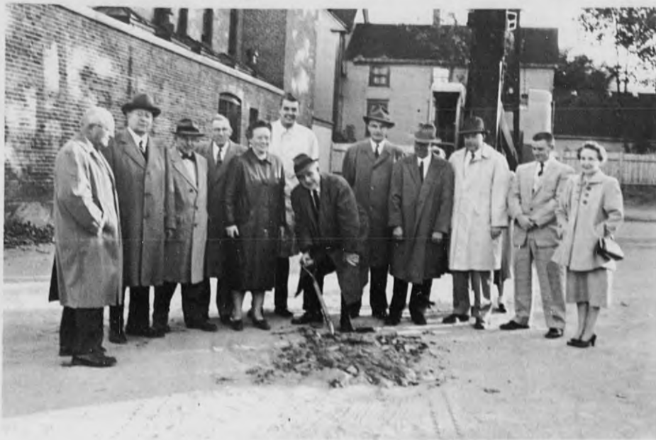
Scene at the ground-breaking ceremonies for the Andover CO-OP's upcoming addition, which took place last Monday morning at 8 o'clock — left to right: Savele Syrjala, Chairman of the CO-OP warehouse; Howell M. Stillman of the Bay State Merchants National Bank; Douglas B. Pitman, Director; Mary Angus, Store Manager; James Carmichael, Director; Winston Blake, President, with spade; Maurice Bailey, Director; Clinton Shaw, Director; Thomas E. Duff, Town Manager; Raymond Fuller, Assistant Store Manager and Catherine Myers, Secretary. Immediately following the ceremony, the power shovel at rear took over and the real digging began.
