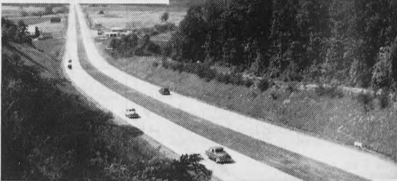
This new-type concrete road is smooth, quiet and comfortable.
