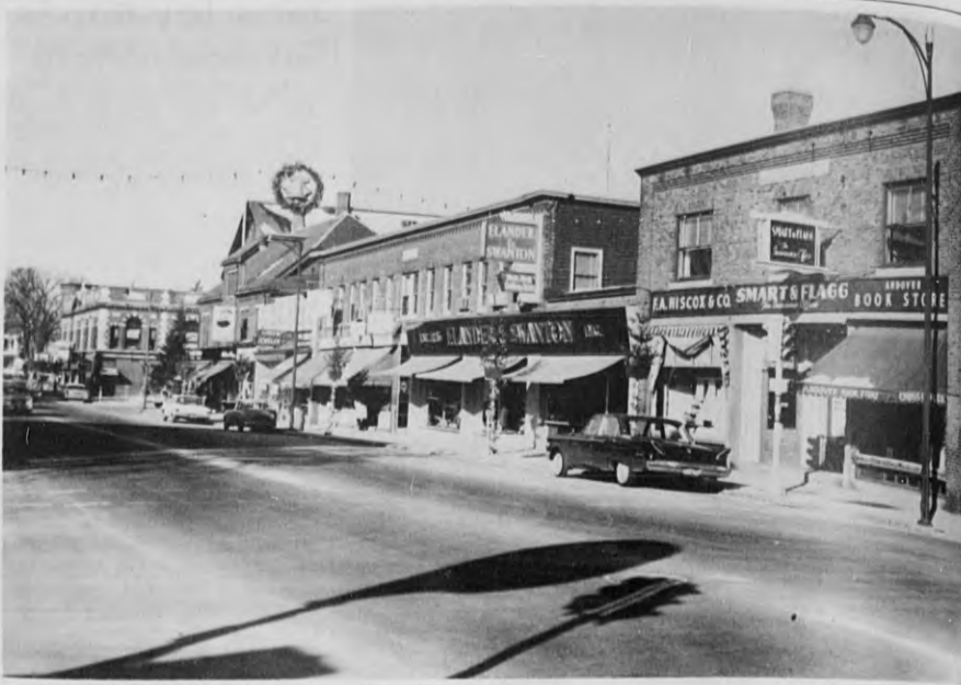
URBAN RENEWAL may radically alter the face of the town's shopping district. This view, taken from Chestnut and Main sts., shows the present easterly side of the street. All of these buildings would be acquired and razed under the present urban renewal plan — over a period of a few years. The decision on urban renewal is expected to produce one of 1962's major debates. (Cole)
