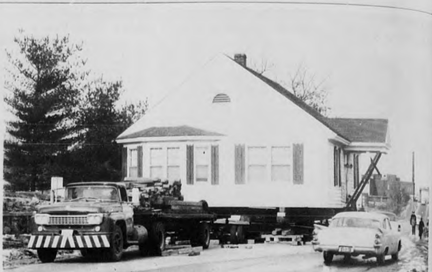
FASCINATING, despite its frequent occurrence, is the profession of house moving. This home was moved from Walker ave. to the new location on Union st., on the last lot before the Lawrence line. One-way traffic moved around the halted house on Union st., as workmen lifted the dwelling high enough to be placed on a foundation on the west side of the street.
