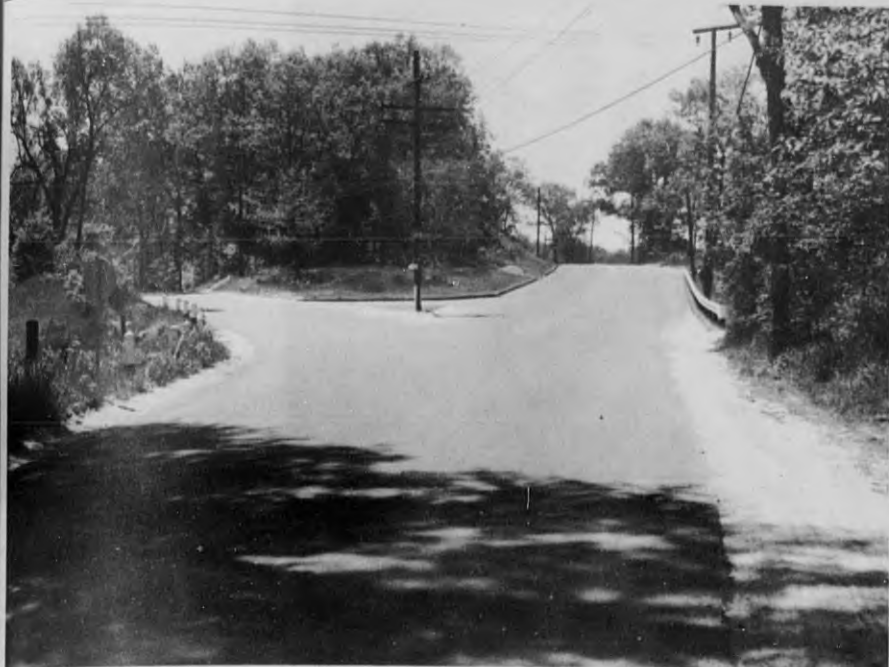
WHAT TO DO? Town Manager Thomas E. Duff, commenting on the intersection of Andover st. and Dascomb rd. - which bears to the right in this photo - said studies are being carried on to determine whether there should be a change in the stop sign. The present signs are on Dascomb rd.; being studied is the possibility of making Andover st. a stop street; or installation of blinking lights. (Staff photo)
