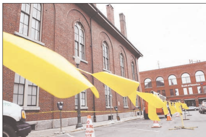
Parking has been blocked off adjacent to Old Town Hall after a shingle fell onto Barnard Street.
