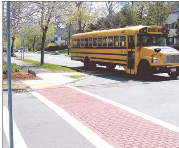
Brick-style crosswalks at the intersection of Whittier and Summer streets are actually made of an asphalt-plastic mixture and are part of the project that created bump-out curbing on Whittier and Chestnut streets.
