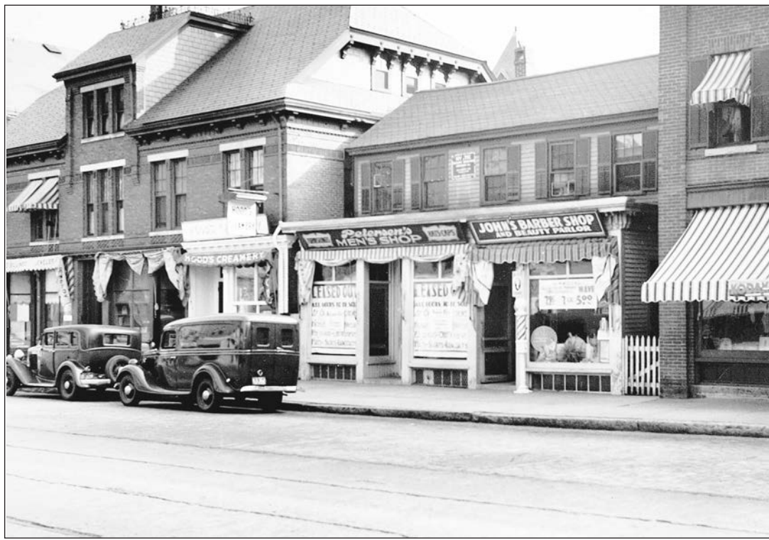
THEN: Around 1936 the building in the center, which housed Petersen's Mens Shop and John's Barber shop, was demolished to make room for the new Woolworth 5 & 10 store. At left was Hood's Creamery and jewelry store.
