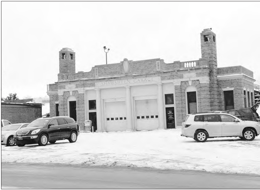
NOW: The garage is now the Woodworth Motors garage.
