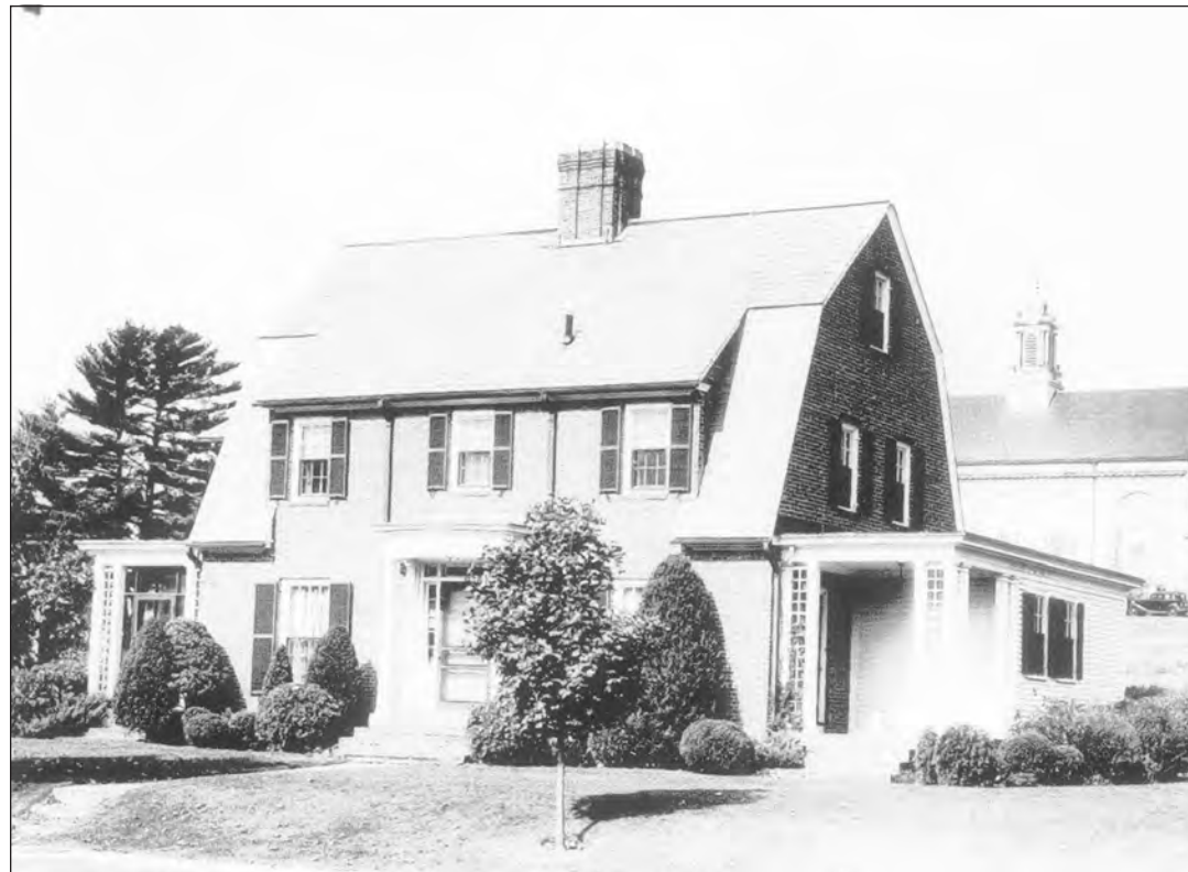
THEN: Developed as housing for the American Woolen Company's executives as part of William Wood's planned community, Shawsheen Village, the homes of "Brick Shawsheen" were placed on the open market by Wood's successor of the company in the mid-1920s, only a few years after they were built. To this day, many still lack a common feature: a garage. Note Shawsheen School to the rear of the home.
