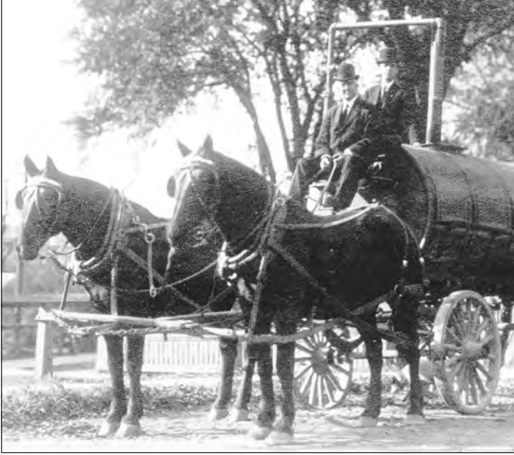
THEN: The water wagon was a familiar sight on Andover's unpaved roads into the 20th century. The horse-drawn wagon continually sprayed the dirt roads with a fine mist to keep dust down.
