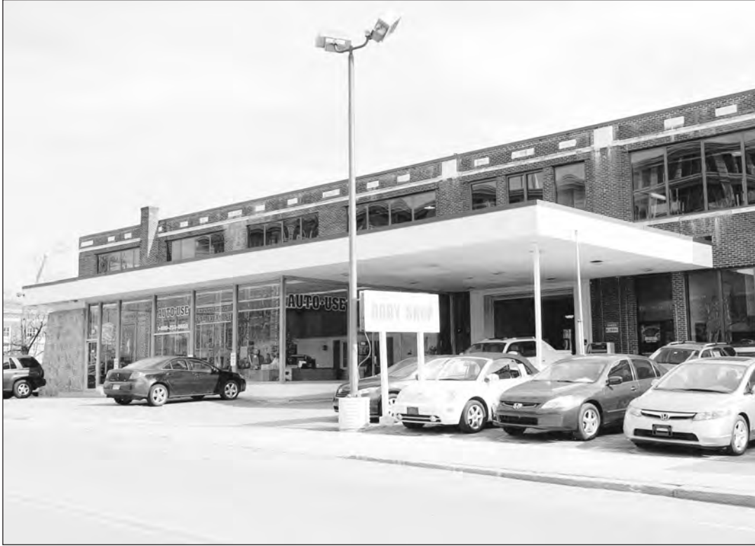
NOW: Still servicing cars, the building is now home to Auto Use.
