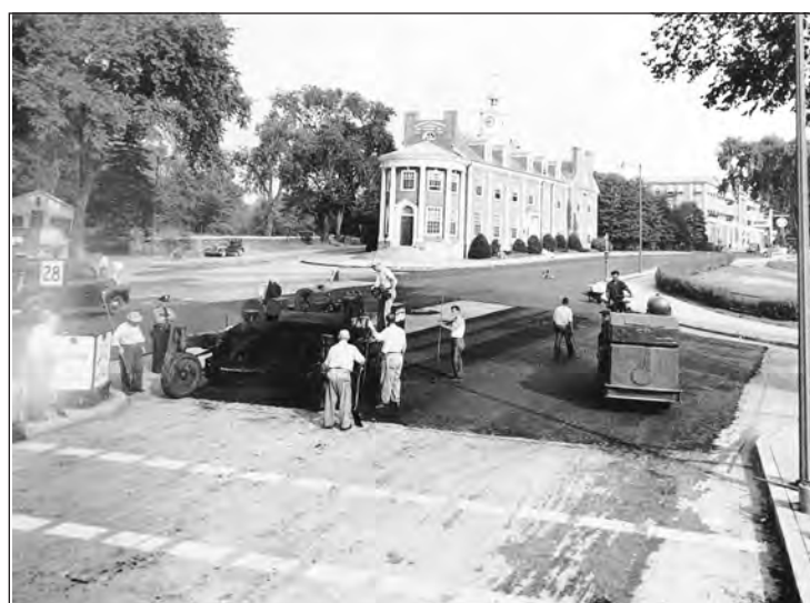
THEN: The intersection of Routes 28 and 133 in Shawsheen Square is paved over with new hot top in about 1950. Police officers would stand in the boxes at left, and direct cars prior to traffic lights being installed.
