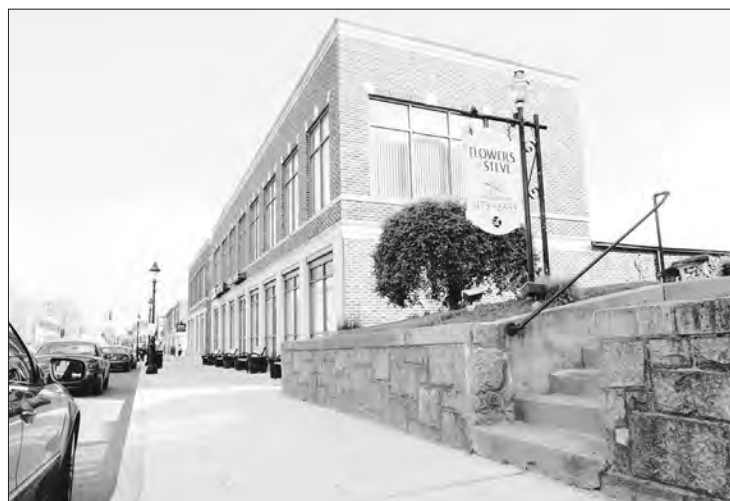
NOW: This is the former location of Barcelos Market on Main Street. While some still miss having a grocery store in the town center, much of the building is now used as a convenience store and pharmacy.
