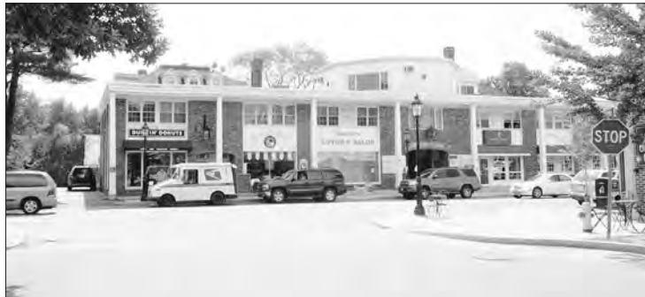
NOW: The roof peaks behind Olde Andover Village are the Homes at 93 and 89 Main St., that were purchased by Lincoln Giles in 1961, and he incorporated them and built around the houses and made the shopping mall.
