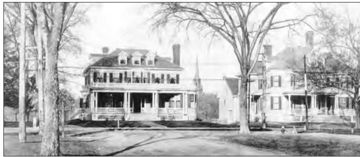
THEN: The Homes at 93 Main St., left, and 89 Main St., were purchased by Lincoln Giles in 1961, and he incorporated them and built around the houses and named it Olde Andover Village.
