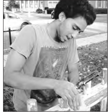
Courtesy photo Andover Youth Services Green Team member Joshua Valentín works on scraping and repainting the fence at Wood Park in Shawsheen this month. Started with a youth employment grant from the state, The AYS Green Team works projects for the town and private citizens, from raking leaves to painting.
