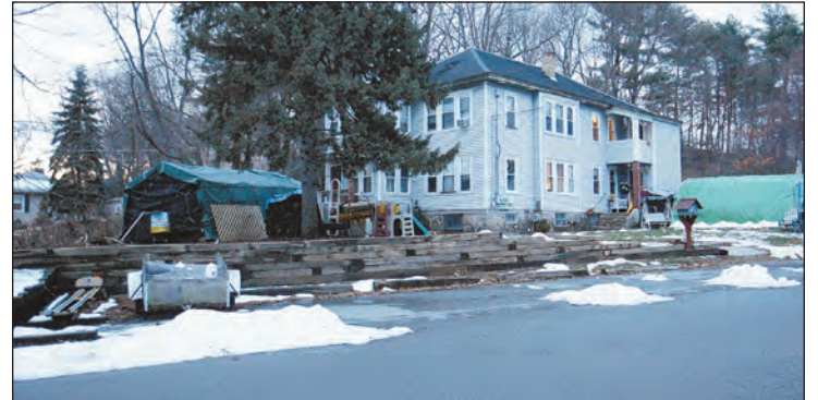
The town of Andover has filed a lawsuit against the residents of 2 Dufton Road because of debris they have left on their lawn.
