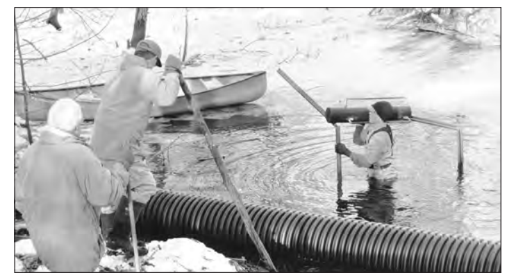
Andover Village Improvement Society trustees, from left, Andy Girdwood, Fred Snell and AVIS Land Manager David Dargie work to install a "beaver deceiver" in the Hammond Reservation.
