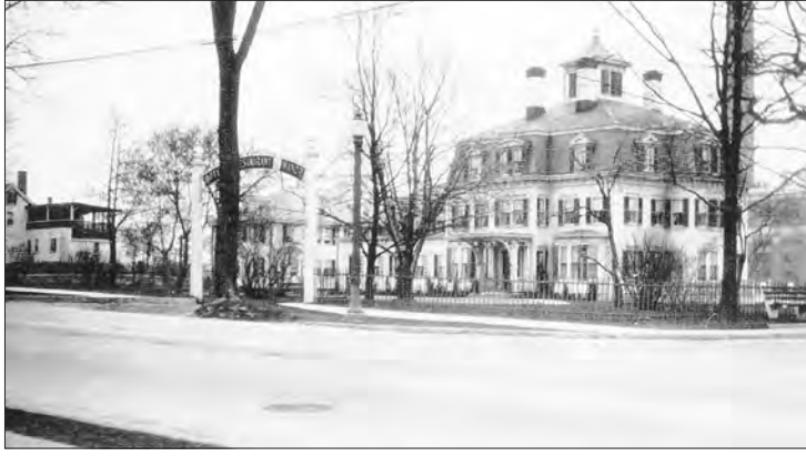
THEN: The Shawsheen Manor on Main Street, was originally the estate of 19th-century mill owner John Smith. It was remodeled and expanded to serve as a hotel for businessmen who traveled to Andover to deal with the Andover Woolen Company. Vendors, agents, and salesman could use telephones for a fee across the street.
