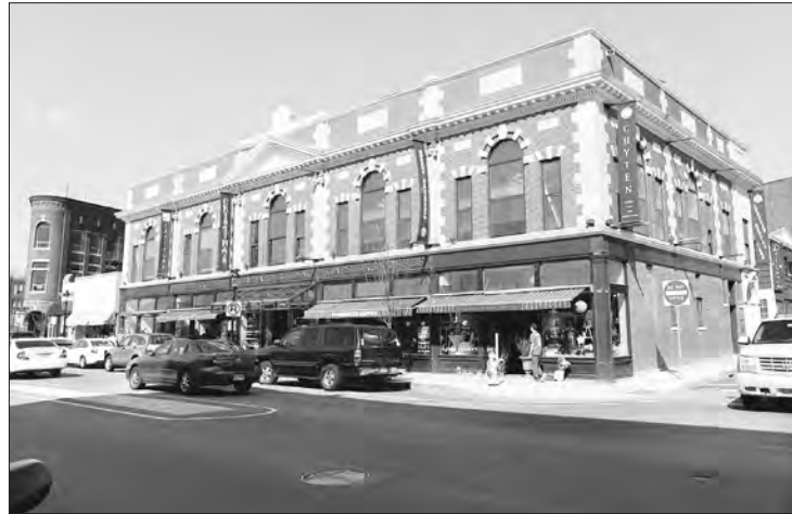
NOW: The intersection of Main and Park Street was home to John P. Wakefield Market and Morrissey stables. The building was leveled in 1910 to build the current building, known as the Barnard Block.
