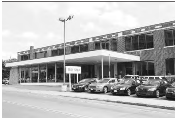
NOW: The site of the former Shawshen Motor Mart on Haverhill Street, Andover.
