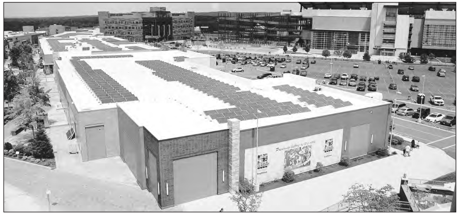
A view of the solar array atop Patriot Place in Foxboro. Gillette Stadium is to the right.
