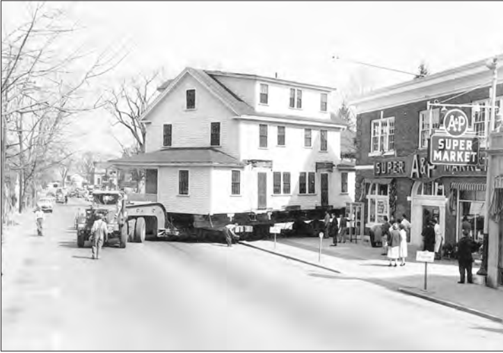
THEN: In May 1955 this 10-room, 80-ton house was moved from 3 Main Street Terrace (behind 84 Main St.) to 150 Main St., making way for a new bank.
