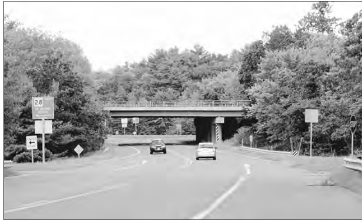
NOW: This is what Route 125 and the Route 28 bridge look like now.
