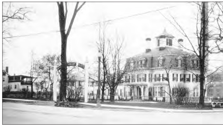
THEN: The Shawsheen Manor on Main Street was originally the estate of 19th-century mill owner John Smith. It was remodeled and expanded to serve as a hotel for businessmen who traveled to Andover to deal with the Andover Woolen Co. Vendors, agents and salesmen could use telephones for a fee across the street. It was demolished in 1989.
