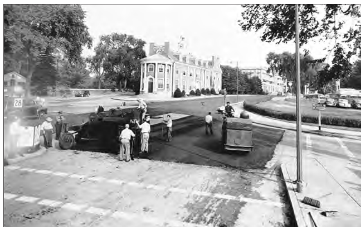
THEN: The intersection of Routes 28 and 133 in Shawsheen Square is paved over with new hot top around 1950. Before traffic lights were installed, police officers would stand in the boxes, at left, and direct cars.
