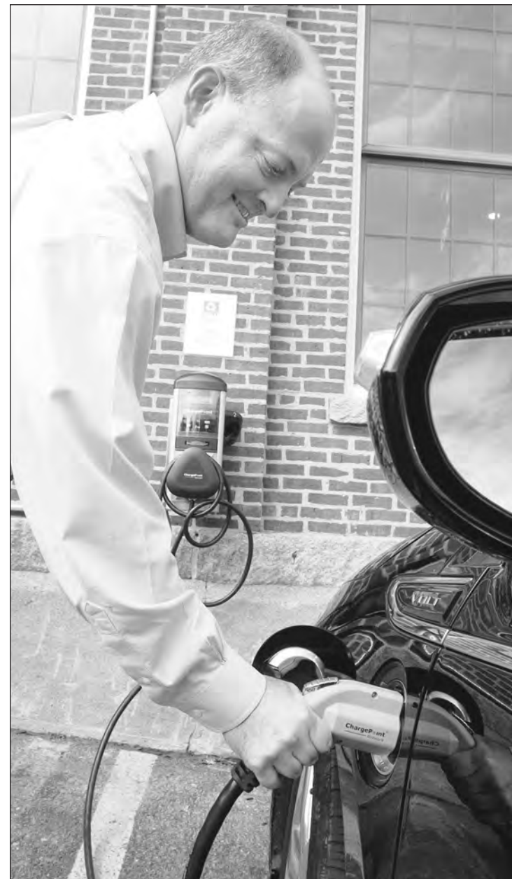
KEN YUSZKUS/Staff photos Tom Wheeler, CFO of EBSCO Publishing in Ipswich, plugs the power cord from an electric vehicle charging station at the company into a Chevy Volt. It is one of two stations at EBSCO.
