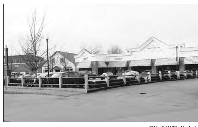
NOW: The parking lot at 34 Park St. was long home to a bowling alley building, the shell of which sat vacant for a few years before it was razed.
