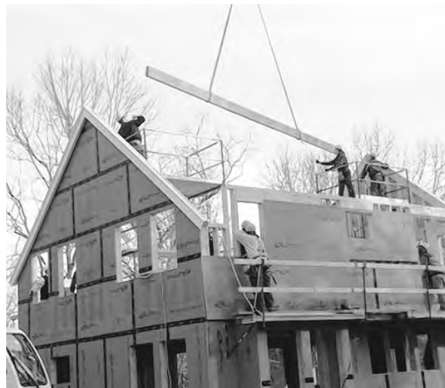
Students and staff of Greater Lawrence Technical School put the ridgepole in place on the Andover Community Trust home they are building on Andover Street.
