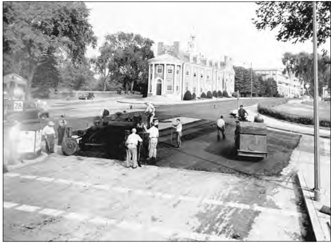
THEN: The intersection of Routes 28 and 133 in Shawsheen Square is paved over with new hot top around 1950. Police officers would stand in the boxes, at left, and direct cars before traffic lights were installed.
